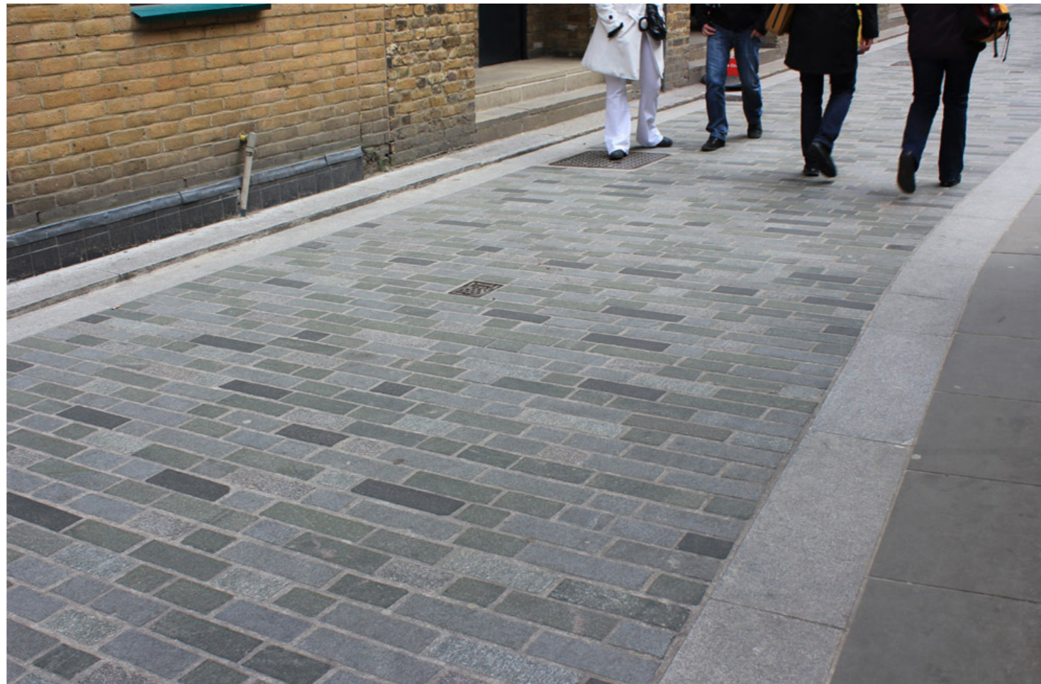
Mixed granite setts, flush kerbs, and footway flags, in shared surface space (Clink Street)
