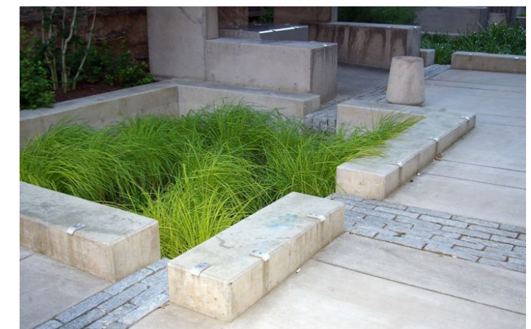
Rain Gardens separated from ground by seating kerb/wall
