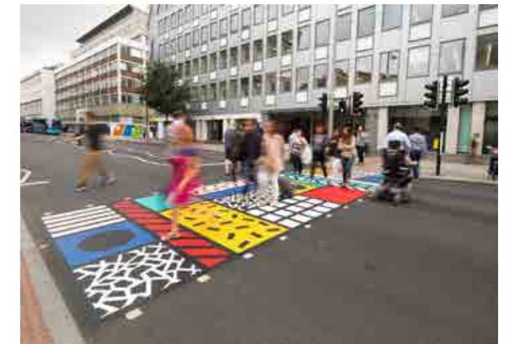
Colourful crossings help to highlight crossing points as well as providing spaces for artistic and creative projects. Coloured crossings could also help with wayfinding by highlighting the Low Line route.
