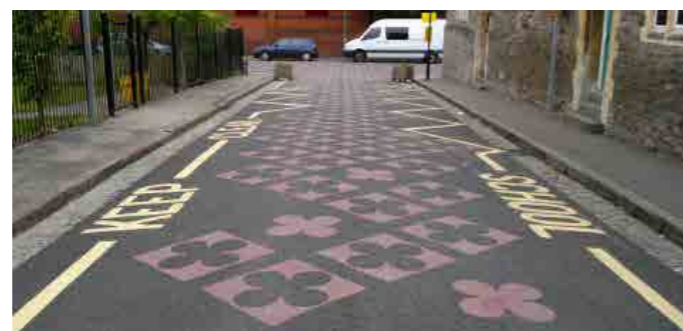
Low tech approach: this example of a school street demonstrates how paint or thermoplastic can be used to create a different surface that indicates that everyone can share the space and pedestrians should be given priority.
