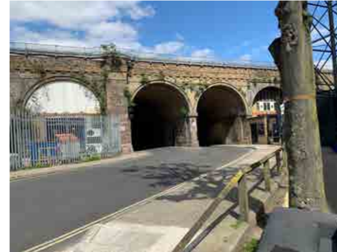
Poor visibility on crossing desire lines
