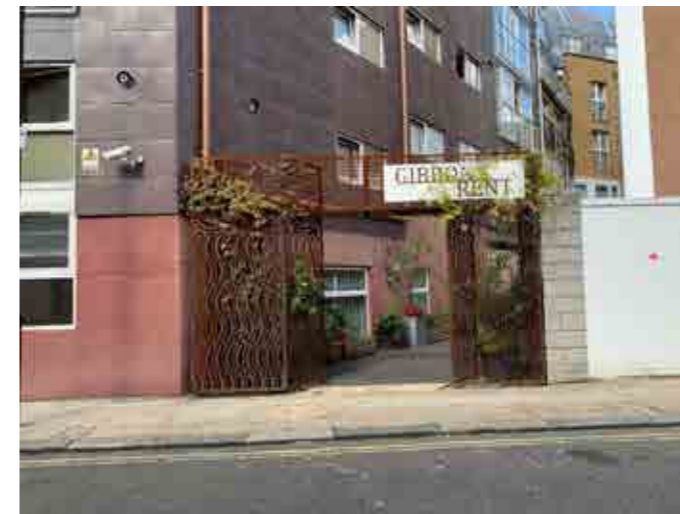
Attractive gateway treatment at Gibbon's Rent in the Holyrood Street area of the Low Line.
