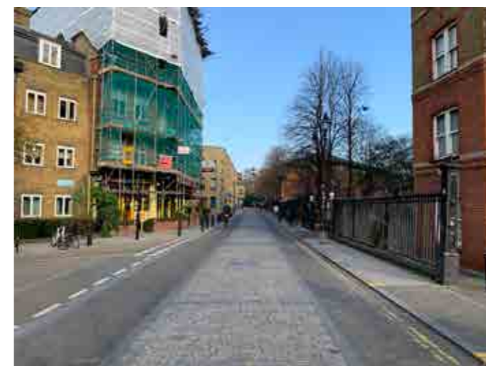
Permanent scheme: Columbia Road in London. The carriageway surface has been raised, leaving only a slight upstand to the footway. The centre of the carriageway has been paved using setts, leaving a smooth concrete block paving on either side to enable cycling.
