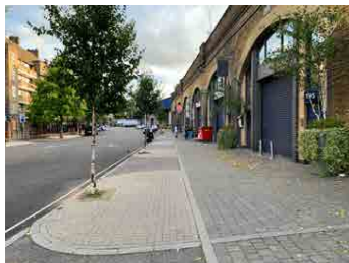
Image: Hercules Road in LB Lambeth, London. Despite the lack of a full height kerb, tree planting and surface treatments help to organise the space, defining a formal footway. The scheme has provided a highquality, safe and accessible pedestrian environment whilst supporting business needs associated with the railway arches, and creating an attractive streetscene.
