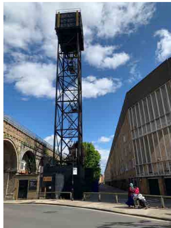
The water tower on Dockley Road/Lucey Way is a distinctive and highly visible feature along the Low Line, however it remains closed off.
