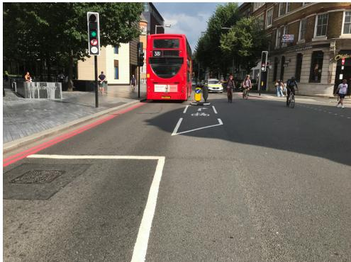
The right turn refuge island has been positioned to leave the eastbound lane approximately 3.0m wide. Emphasis should be given to the cycle route by placing pairs of Diag 1057 cycle logos centrally in the lane.
